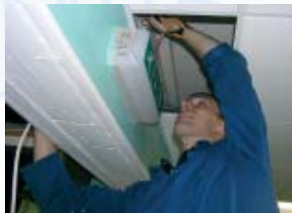
Andy Ethel works on the lighting circuit
